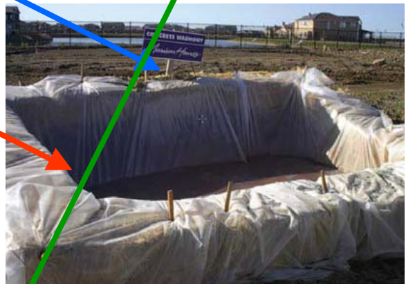
Designated Concrete Washout Containment Areas
