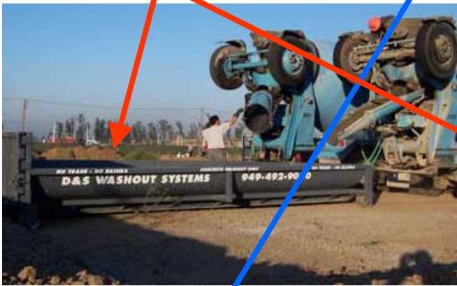
Designated Concrete Washout Bin
