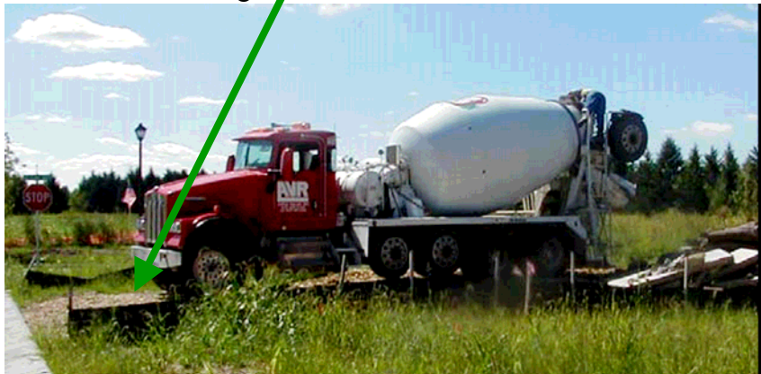
Designated Concrete Washout Bin
